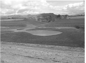
Fig. 14: View of the reservoir from the west showing the 'V' notch, pools and embankments formed in the reservoir basin.
