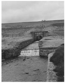
Fig 7: Masonry step overflow weir
